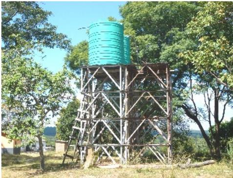
The water tower at the Home is currently being repaired. Two of the four tanks have had leaks which have been mended, and the wooden platform on which they sit is being renovated with new timber. Once the new generator is installed this tower will be important in re-establishing running water in the main house.
