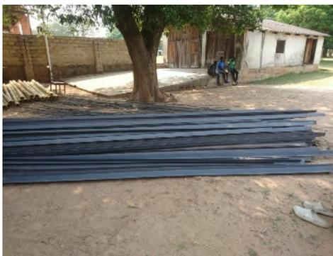
*Steel for making the roof trusses*
