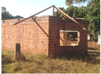
The new toilet block
